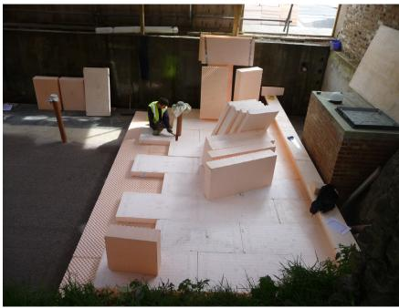
(above) The Isoquick insulated foundation system eliminates any thermal bridges between the floor and walls; (Top right) while the lower level is built in reinforced concrete, the cross-laminated timber panels are also used for partition walls; (Top left) excavation works were carried out and a retaining wall constructed as local planning rules required the house to be set half a level down from the street
