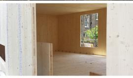
(above) The upper level is constructed with crosslaminated timber panels, which is a more flexible way of prefabricating with fewer materials involved and allows for simple assembly. The large building elements involved also mean fewer joints, which means less likelihood of air leakage, improving the airtightness of the building
